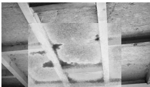
Figure 1: Moisture in the ceiling structure
