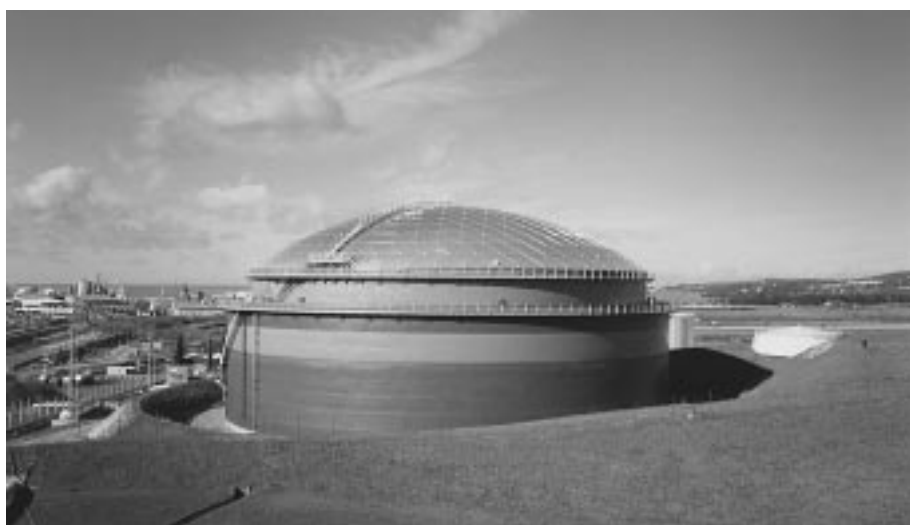
Slika 10: Rezervoar v obratovanju Figure 10: Collecting tank in operation
