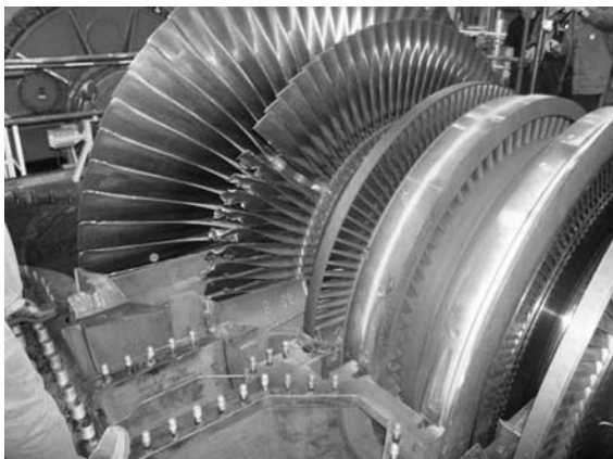
Figure 1: Damage to the 3TW on the TG1 Slika 1: Poškodba 3TW na TG 1
